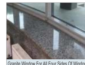
Granite Window For All Four Sides Of Window
